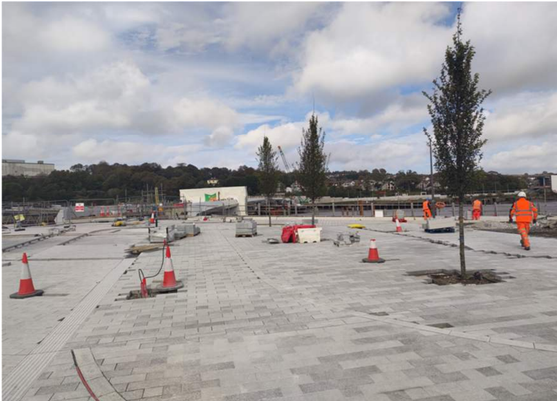
Figure 14 Construction Underway of South Plaza Oct 2025
